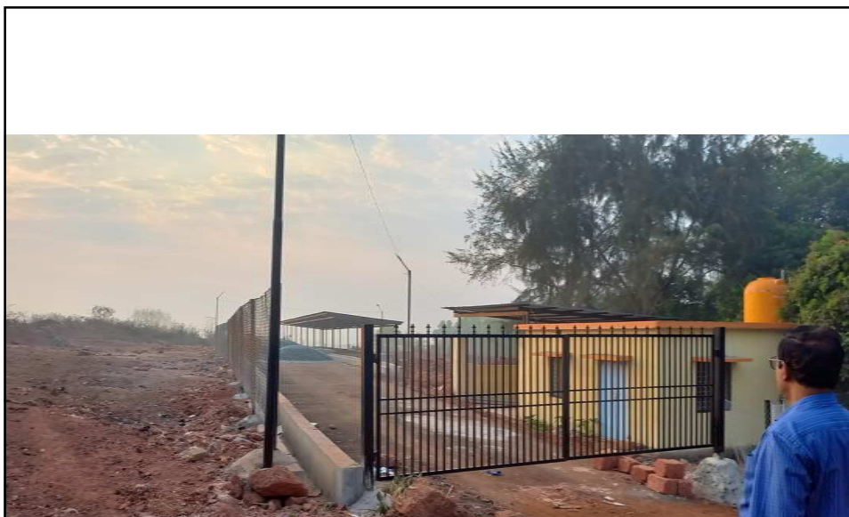
New site where GP Gokarna established fecal sludge treatment plant.
